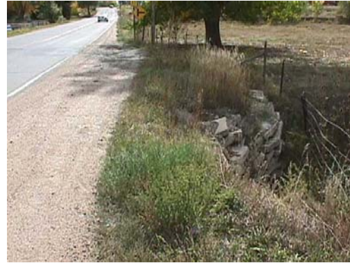
Van Bibber Creek Bridge
