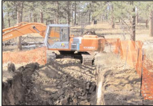
Septic system excavation
