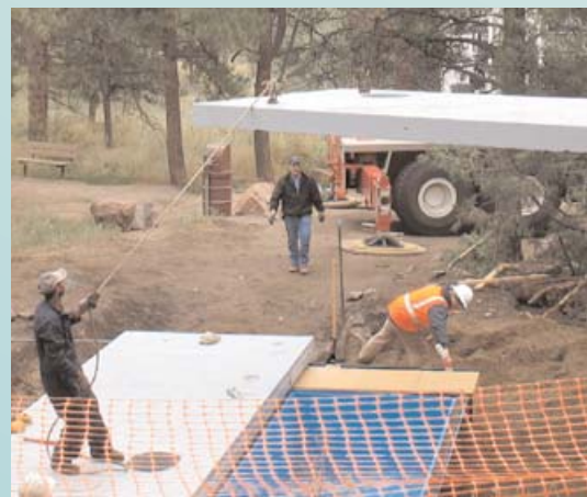
Construction of a new restroom at Alderfer/Three Sisters Park.
