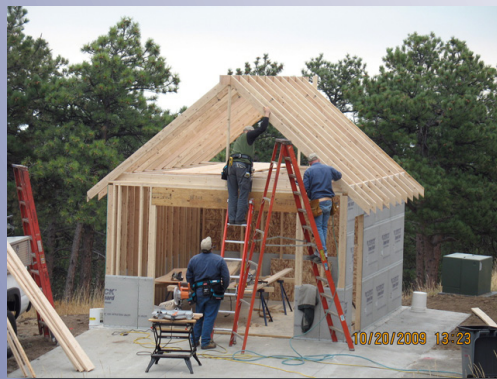
Lookout Mountain Nature Center's storage shed construction.
