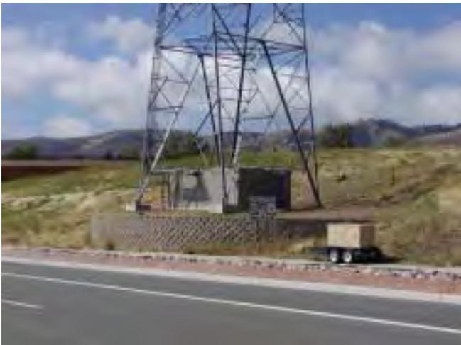
Panels match the industrial appearance of the transmission tower and by virtue of their relative size and coloring, are rendered unnoticeable. Equipment enclosure façade matches the brick of the retaining wall. Small dish antenna should be painted gray, but otherwise this installation should qualify as HDS.
