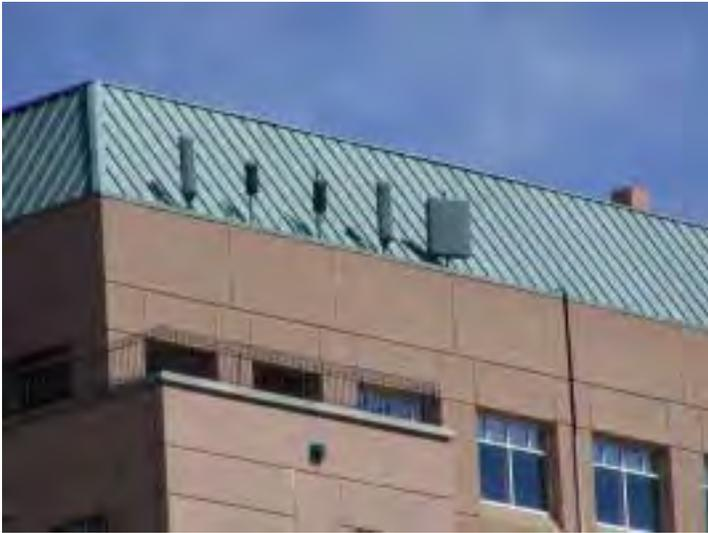
Acceptable as general roof mount, but should not qualify as HDS. Better if mounted on the face of the building or installed behind RF translucent screening.
