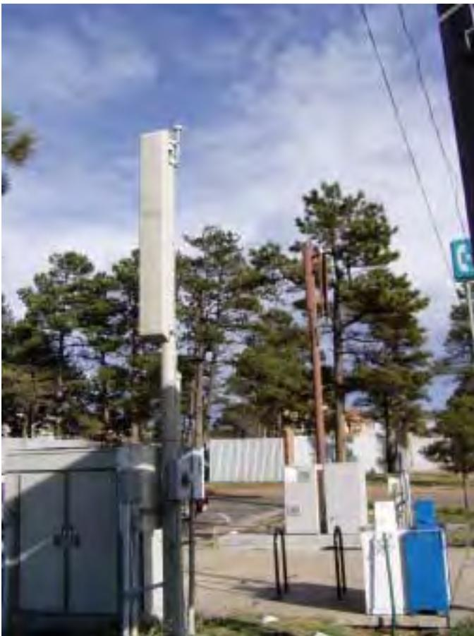
Good location, but this is an example of too many facilities in one location causing the entire site to become visually obtrusive. Situation could be improved by integrating antennas with light poles and screening or burying equipment boxes.
