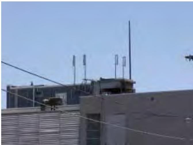
photos demonstrate poor examples of roof mounted facilities. Screening or integrated construction necessary for standard roof mount. Building mounted panels in middle photo should be smaller and painted to match the building.
