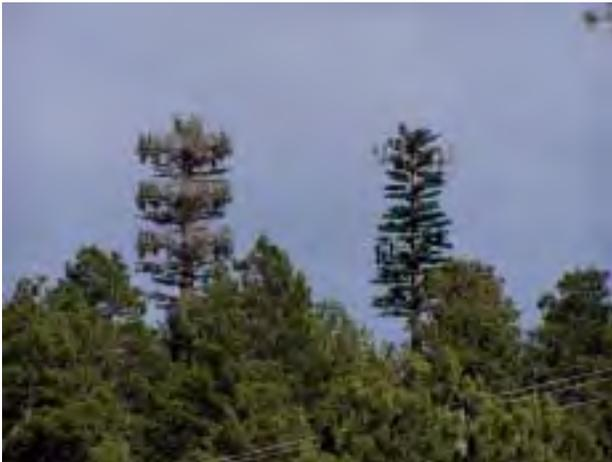
Top and Middle: Good example. “Tree” is in scale with surrounding trees (generally equal in height with the tree line). Would be even better if antennas were internal to the canopy.
