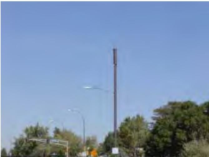
Top: Excellent example of light pole application for use in all rights of way. Panel is flush mounted painted to match and keeps the light pole in scale .
