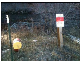
Figure 1. Drafting point (dry hydrant) near Longview
